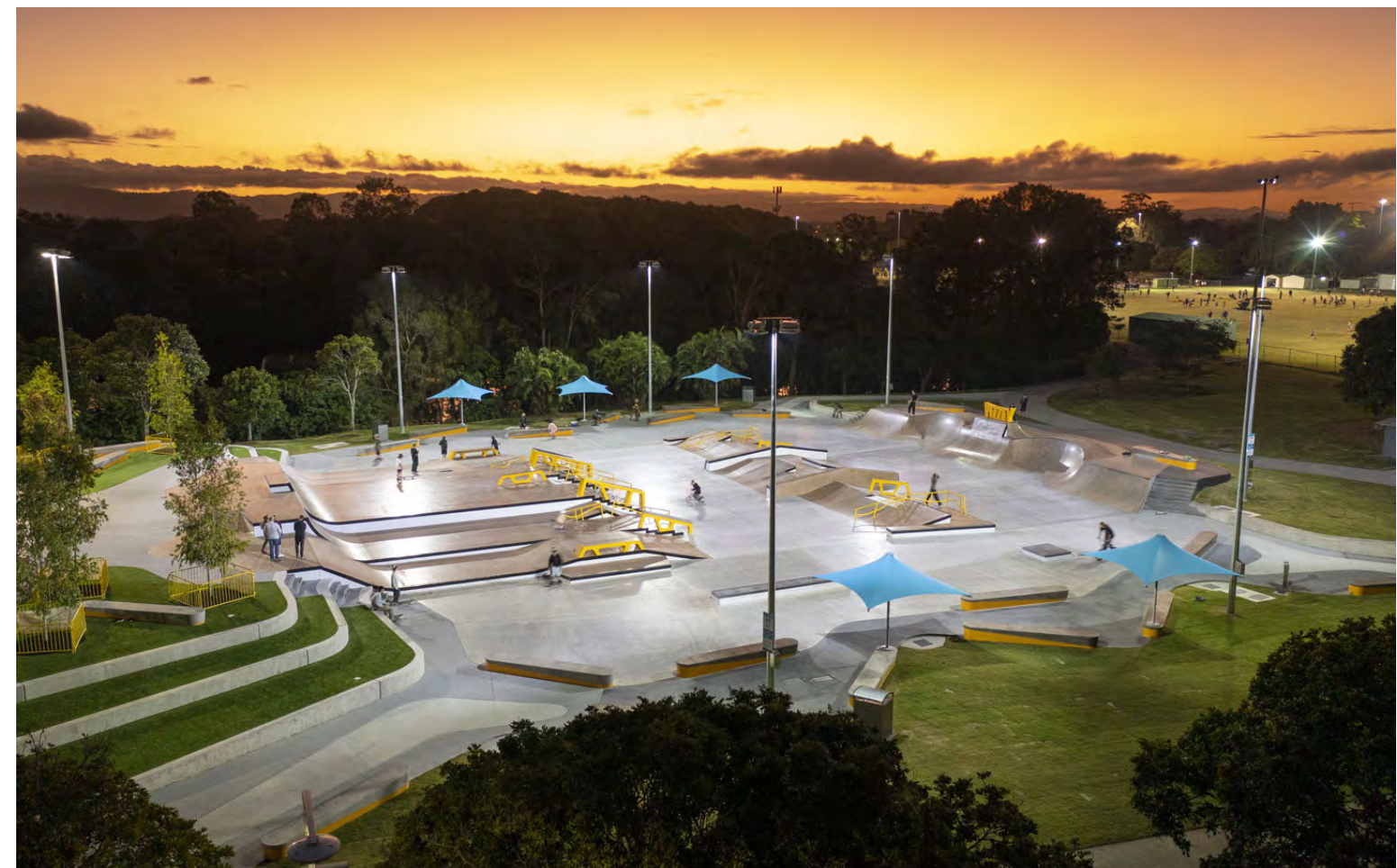
Fig. 8. Overhead shot of Pizzey Park Skate Park in Miami, Queensland from: Schreder "Pizzey Park Skate Park." 2022.
