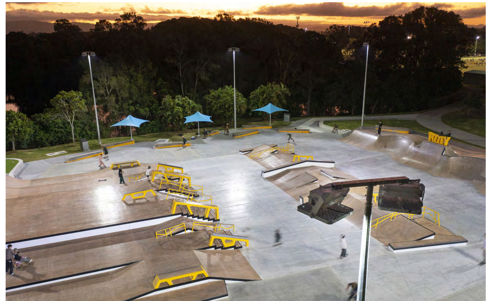
Fig. 7. Overhead shot of Pizzey Park Skate Park in Miami, Queensland from: Schreder "Pizzey Park Skate Park." 2022.
