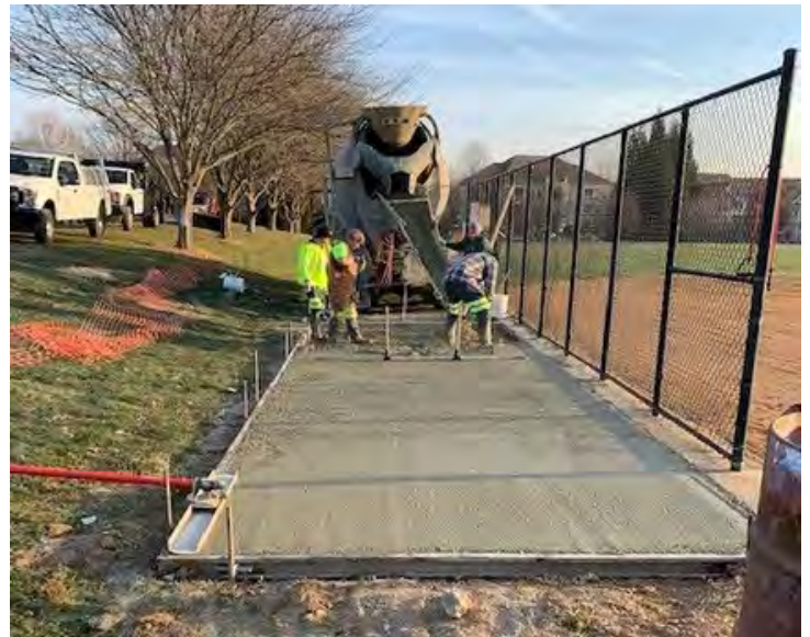
(Left) An example of a blue stone player's bench area that can be prone to weeds. (Right) A poured concrete player's bench area is installed at Fountain Hills Local Park to allow for easier maintenance.
