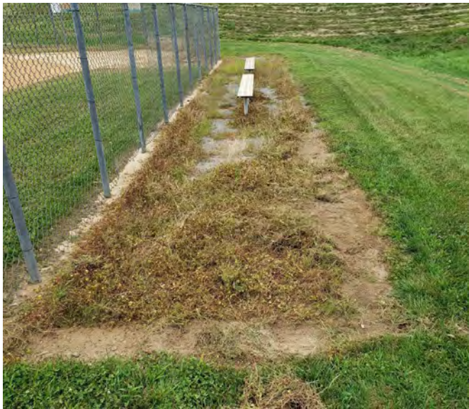
(Left) An example of a blue stone player's bench area that can be prone to weeds. (Right) A poured concrete player's bench area is installed at Fountain Hills Local Park to allow for easier maintenance.
