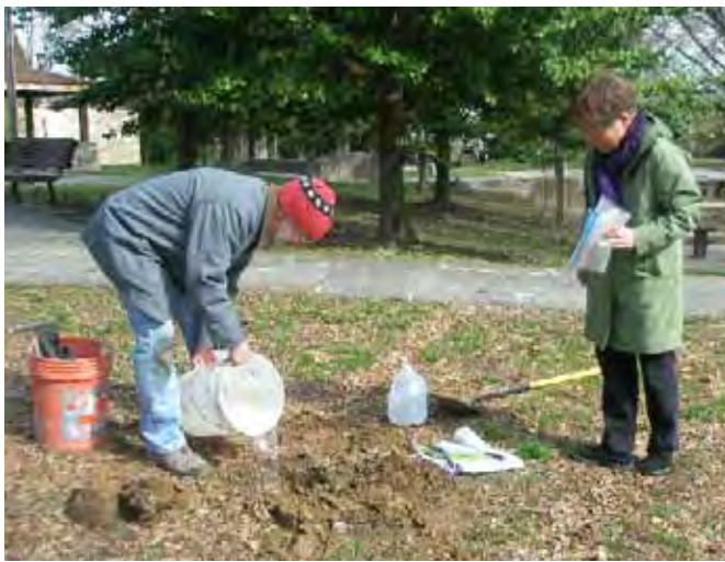
^ Field Percolation Test 1
