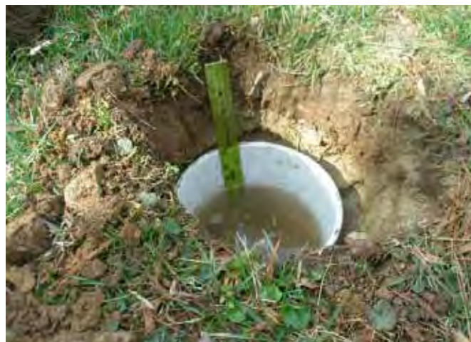
^ Field Percolation Test 2
