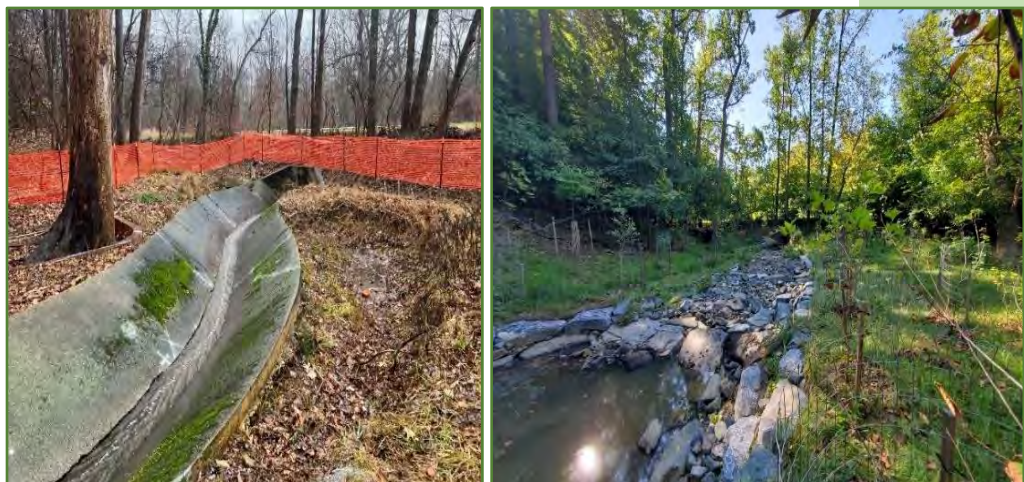
Wildwood Road Outfall pre-construction (left) and post-construction (right).
