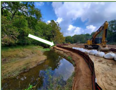
Proper erosion and sediment control practices installed on a construction site.
