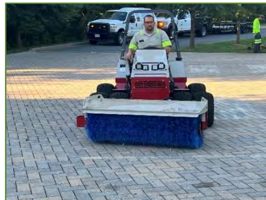
Water Quality Staff perform maintenance on pervious pavement.
