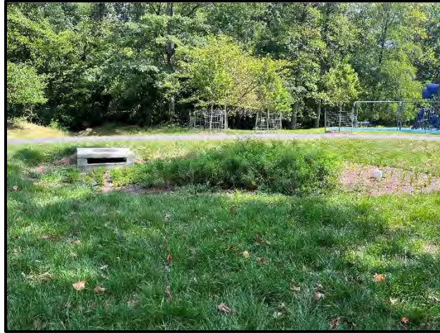
Above picture: Dale Drive Local Park Bioretention
